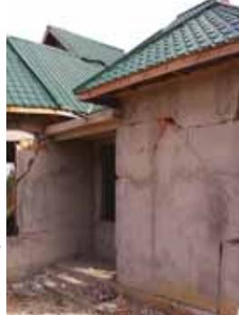
A single storey unsymmetrical building (with accessible roof balcony), of height 4 m with some gable partition walls experienced major failure due to Kagera Earthquake.
